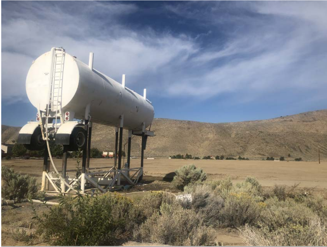
Photo 3: Water Tank Along the Eastern Edge of the Site
